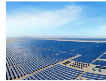
Photovoltaic power station
