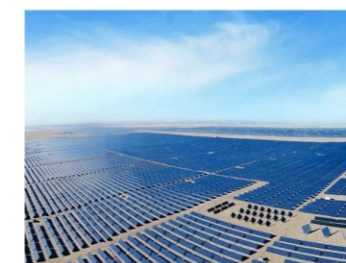
Photovoltaic power station
