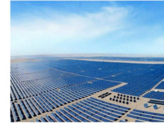
Photovoltaic power station
