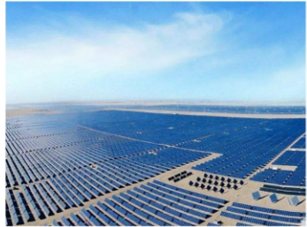
Photovoltaic power station
