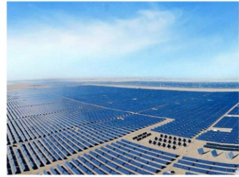
Photovoltaic power station
